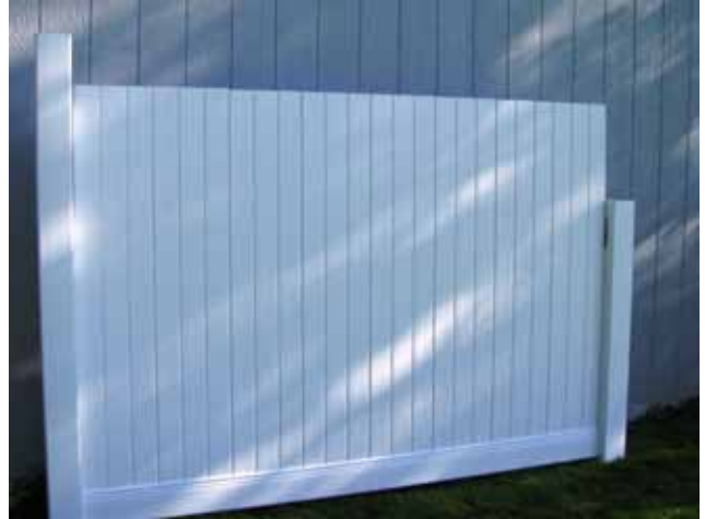
2. Insert Pickets in Bottom Rail
